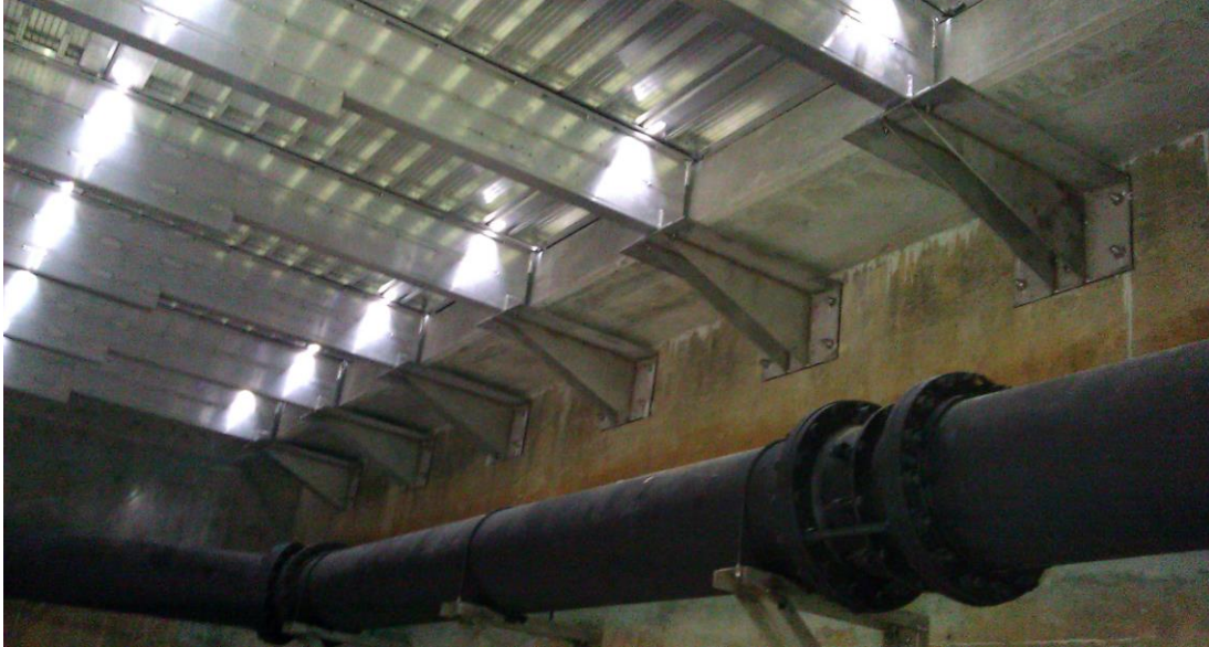
Figure 6.8 Cover Mounting Brackets
